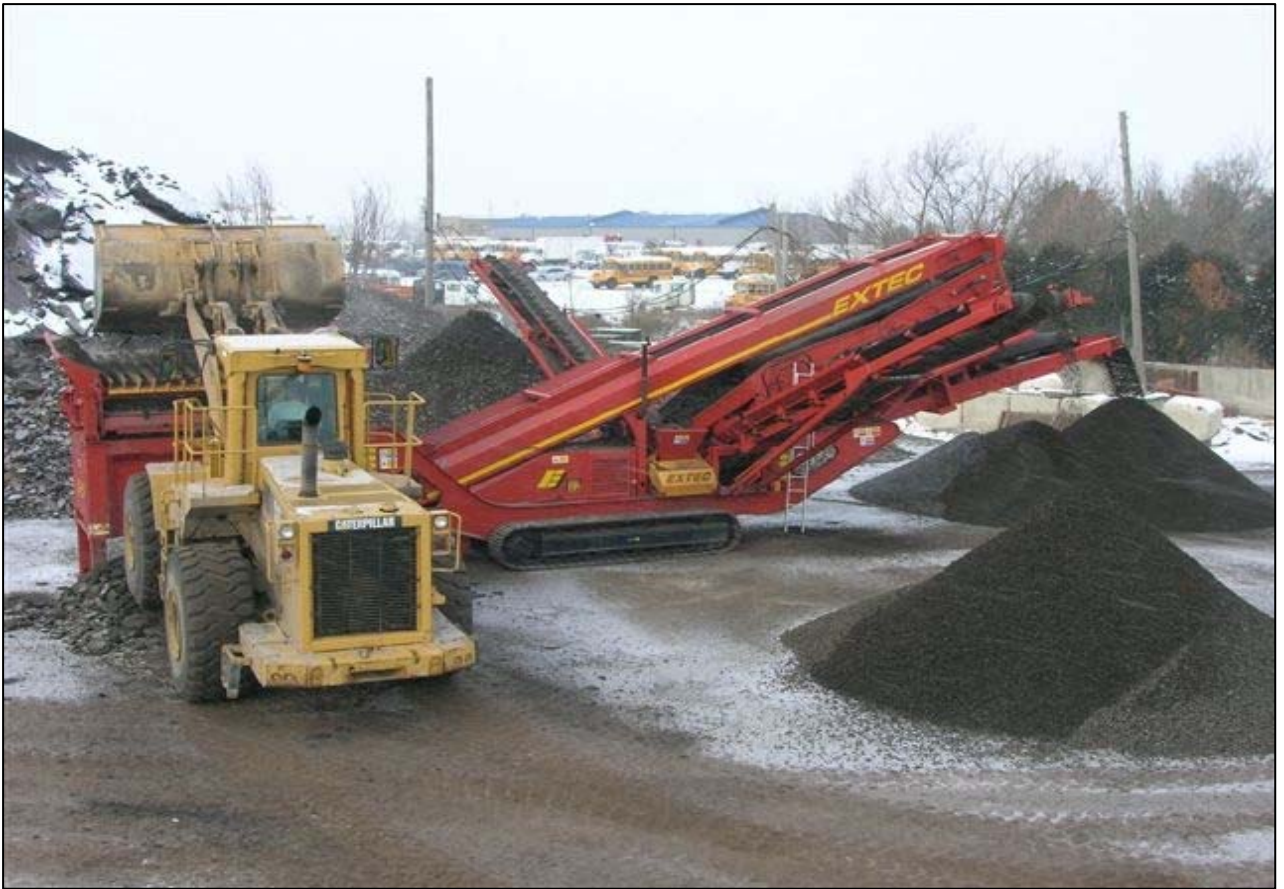
Asphalt millings application
